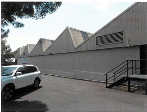
Figure 6: Current view of the Shepherd Street facade showing the replacement wall and roofing materials
