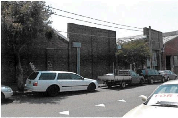
Figure 14: View, looking east, showing the eastern end of the heritage listed facade
