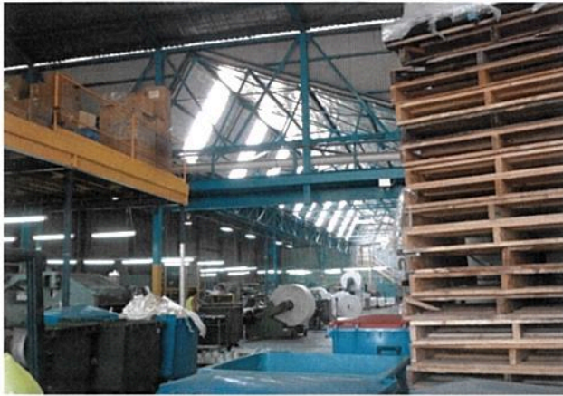
Figure 8: The junction of the rear extension and the original factory structure, looking west, showing the rear wall of the factory was removed
