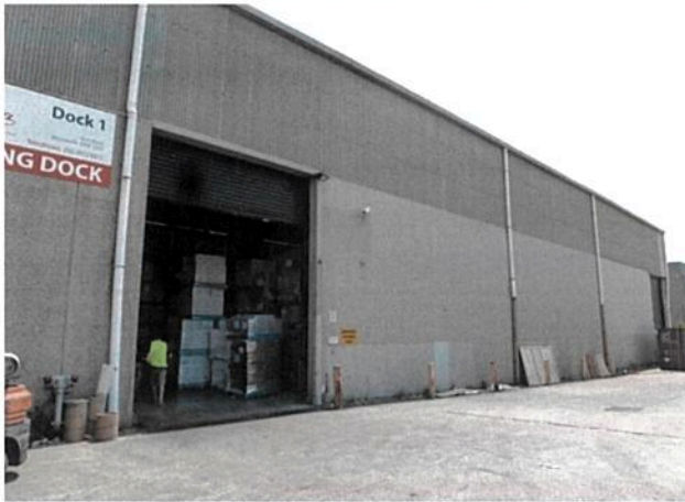
Figure 9: Rear (east) facade of the factory extension, at the end of Rich Street
