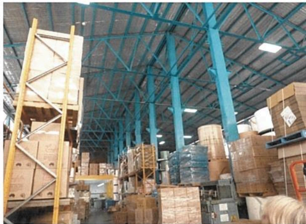
Figure 10: Photograph of the interior of the eastern addition showing the simpler roof structure
