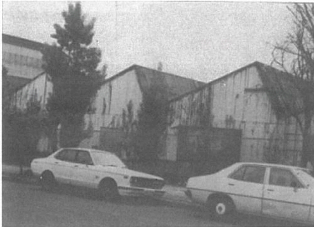
Figure 5: 1984 photograph of the Shepherd Street (west) facade of the factory showing the earlier corrugated iron cladding that was identified as being of heritage interest
