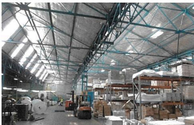
Figure 7: Interior of the factory building, looking west towards Shepherd Street, showing the saw tooth roof structure
