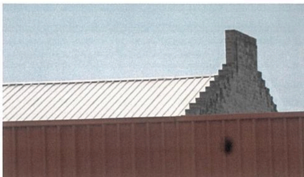
Figure 11: Brick gable to the party wall at the southern end of the post 1943 eastern addition to the factory at 61-65 Shepherd Street
